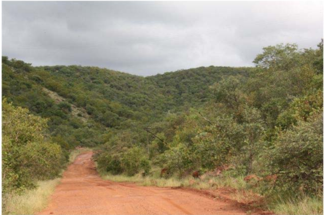
VIEW C: VIEW FROM LOCAL ROAD TOWARDS ALTERNATIVE B COMING DOWN THE NECK
